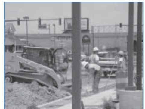
Work being done on Lewis & Clark Parkway.
