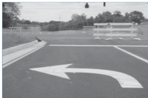
Construction is almost complete on Hurstbourne extension.
