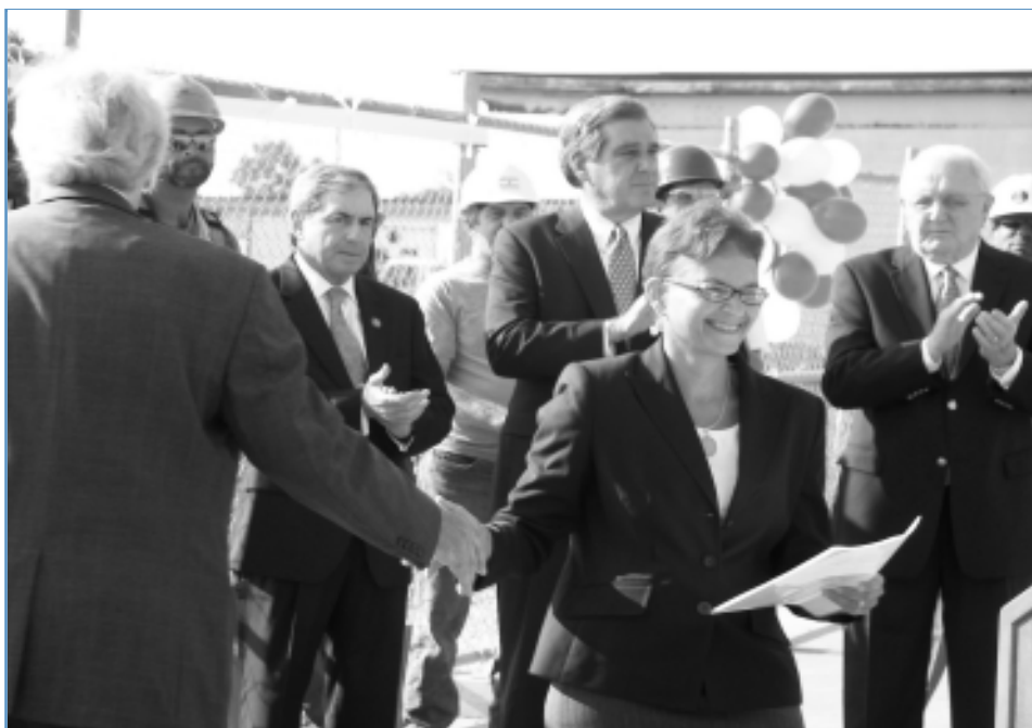
TARC broke ground on its Maintenance Annex Building on August 25. The project is expected to create 80 jobs.
