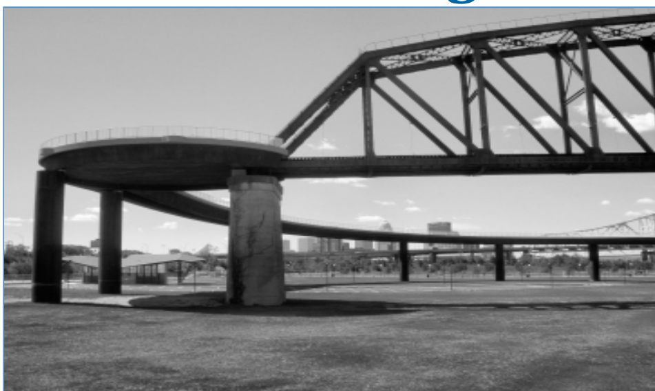
The ramp leading up to the Kentucky side of the bridge has been completed. Photo courtesy of The Waterfront Development Corporation.
