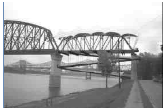
View of the Big Four Bridge from Mulberry Street in Jeffersonville.
