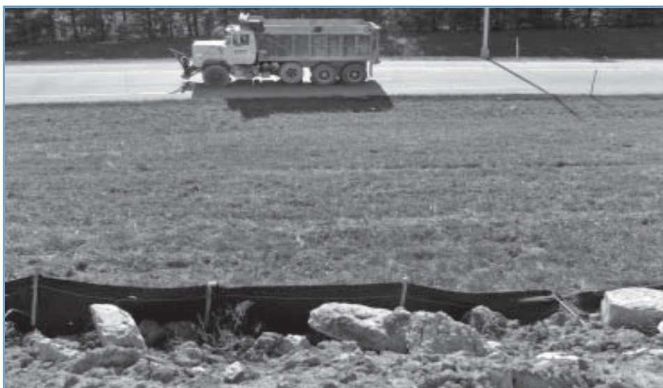
Work is underway on the Bardstown Road exit ramp.
